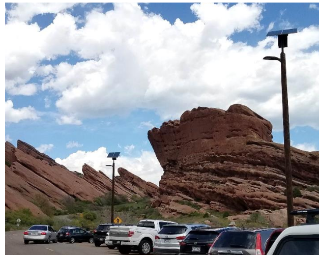
Figure 32: Solar Lighting Installation
