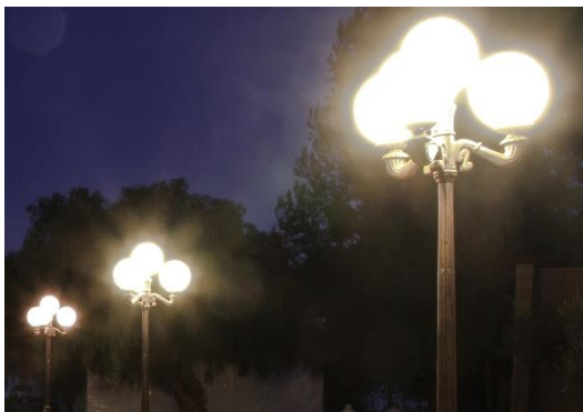
Figure 48: Reduce Glare with Appropriate Luminaires
