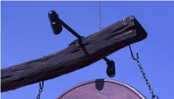
Figure 39: Example of a Small Floodlight Oriented Downward
